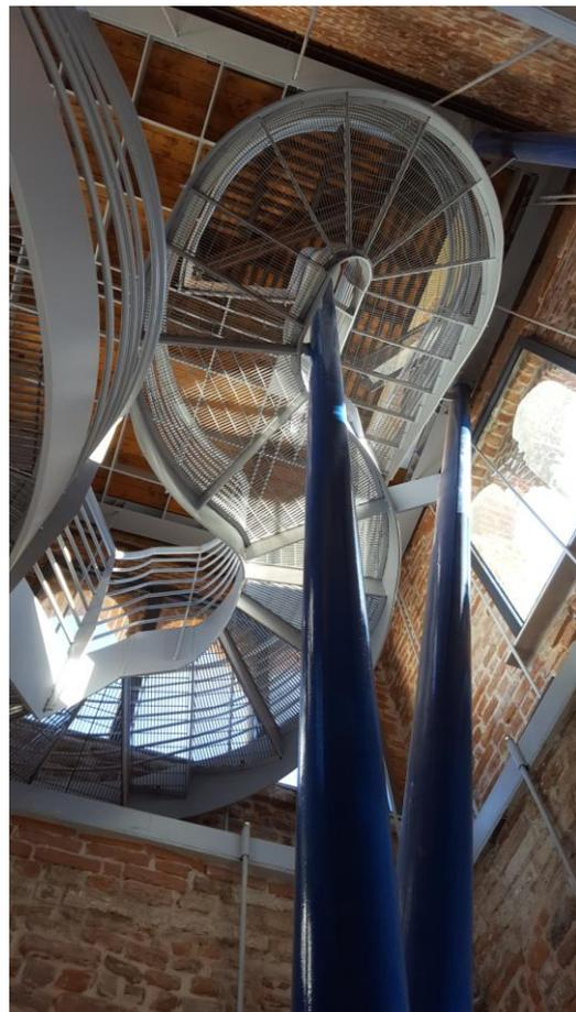
*Fig. 3. The new steel stair in Gorani Tower*
