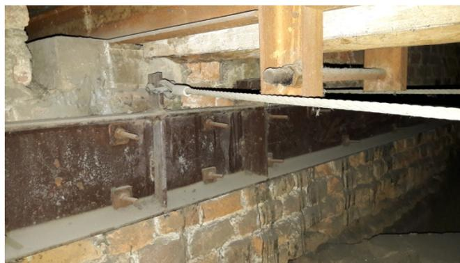
Fig. 3. (a) FE Model implemented in 1980s to determine the cause of the crack pattern through a “back analysis”; (b) “C” shape steel element and bracing structures introduced in 1980’s
